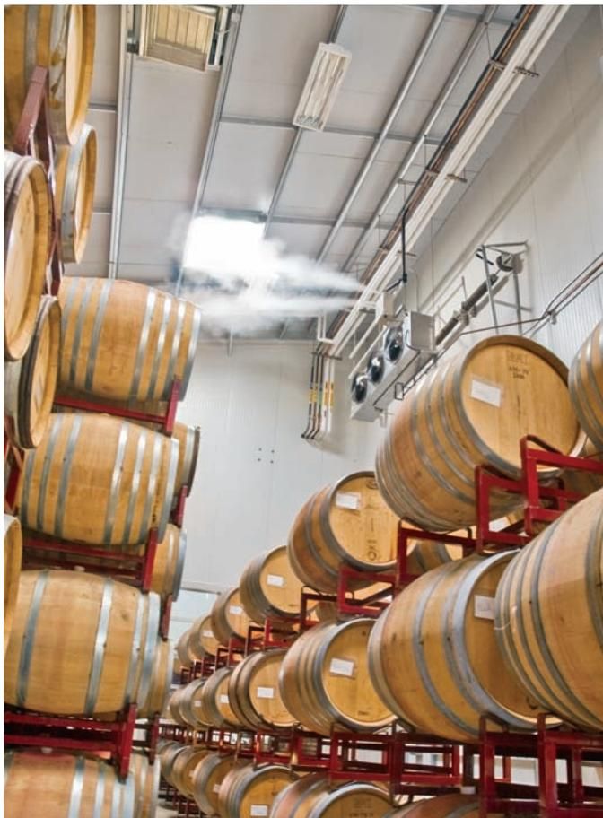
Smart Fog in each barrel room is programmed for 10-second dispersal every 30 seconds. System activates within 2% of setpoint (75% humidity).
