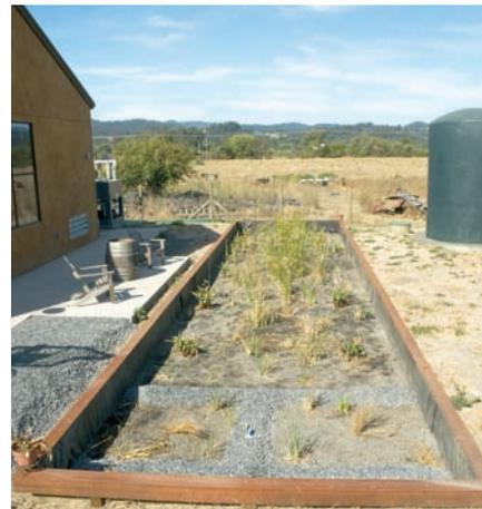
**The constructed wetland was designed to enhance the site as a landscape feature and provide a system to allow the reuse of treated wastewater.**
