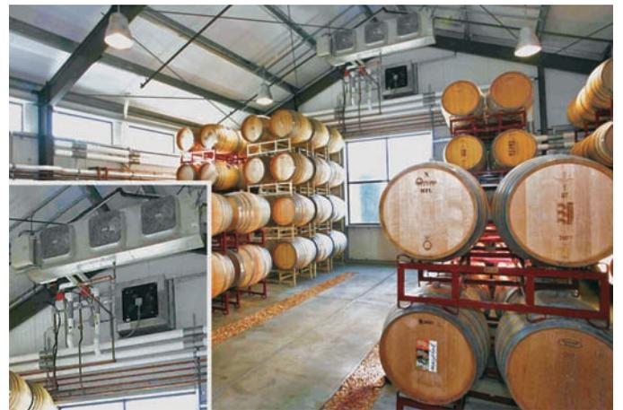
Maximum capacity of the barrel room is 300 barrels. Between the rows of barrels are gravel-filled drain-trenches. Inset: Night-cooling fans and Smart Fog ES 100 humidifier.
